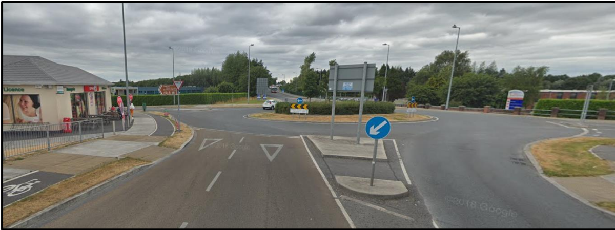
Figure 3.5 – Approach to R916/Moydrum Road roundabout from the south (Source: Google Maps)
