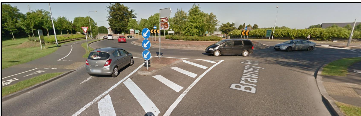
Figure 3.7 – View of Brawney Road approach to R915/N55 roundabout (Source: Google maps)
