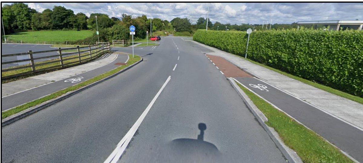
Figure 3.4 – Existing infrastructure at Blackberry Lane (Source: Google Maps)
