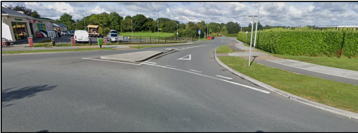
Figure 3.6 – View of Blackberry Lane approach to the junction (Source: Google Maps)
